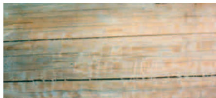
Felted wood after power washing.
